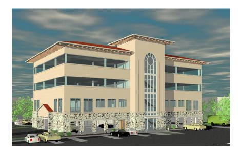
The building consists of three floors of medical office space over a level of parking, and is the third in a series of three medical office buildings on the site. Design requirements included matching the two existing buildings in terms of materials and general concepts, as well as conformance with existing civil sitework and utilities which were already in-place on the site.
